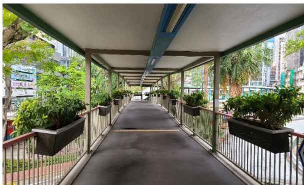
Railing Planters on Footbridge
